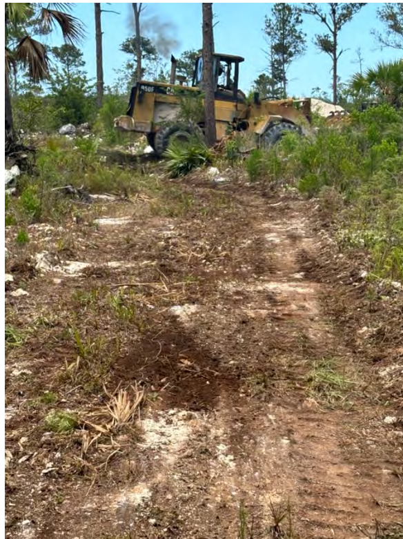
Bulldozer actively clearing the site
